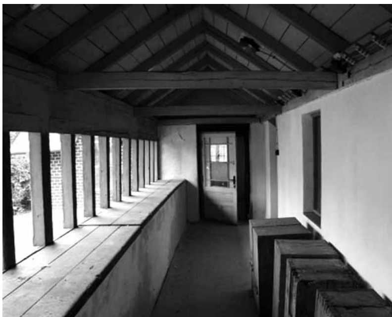
Fig. 3 The bee room inside with the old hives (right), all is waiting for conservation and renovation
